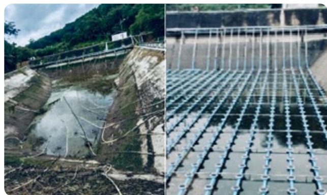
1 Before : 105 diffusers BOD: 446, TKN: 728 After : 523 diffusers BOD: 34, TKN: 45
